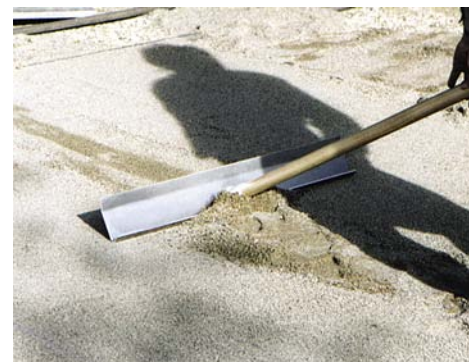
Figures 5 and 6. After removing screed rails, the voids are filled with sand and smoothed with a trowel or a flat rake sometimes called a "come-along."
