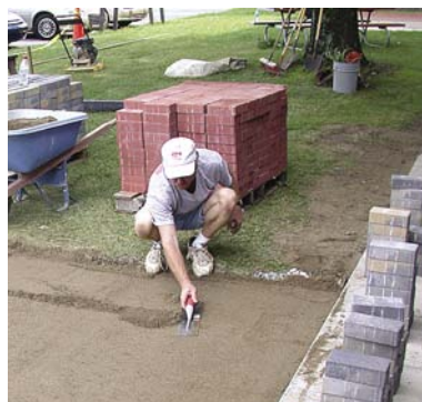
Figures 5 and 6. After removing screed rails, the voids are filled with sand and smoothed with a trowel or a flat rake sometimes called a "come-along."
