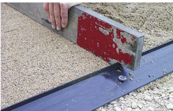
Figure 4. A notched screed board easily rides along plastic or metal edge restraints or curbs.
