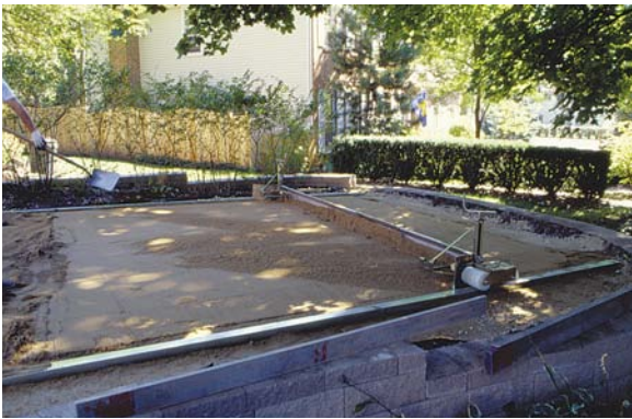
Figure 2. A mechanical screed is useful for doing straight driveways and other large areas. Most designs can adjust to various lengths.
