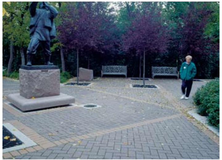
Figure 5. Incorporating banding and a change of direction can reduce cutting when paving around an obstruction.
