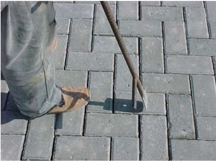
Figure 4. An alignment bar, shown above adjusts joint widths to maintain bond lines.
