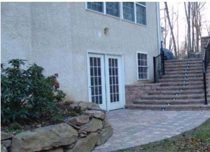
Figure 7. Finished view of steps
