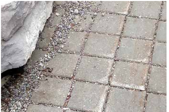
Figure 15. Coarse debris like winter sand should be removed from the paver surface to reduce abrasion.
