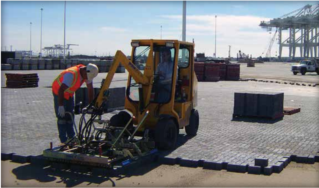
Figure 8. Mechanical installation equipment places concrete pavers rapidly.
