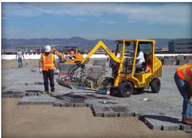
Figure 5. Motorized equipment with a hydraulic clamp.
