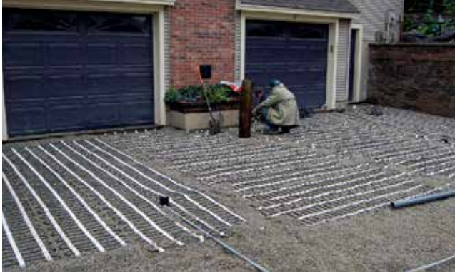
Figure 10. Electric heat tape snow melt system is installed in the bedding layer of permeable interlocking concrete pavement.
