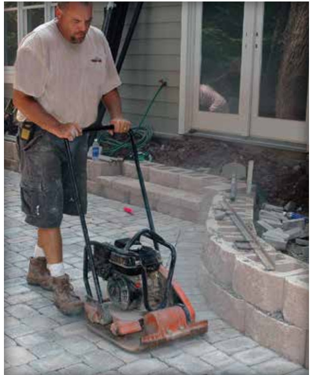
Figure 9. Final compaction of the pavers and settling of the sand into the joints.
