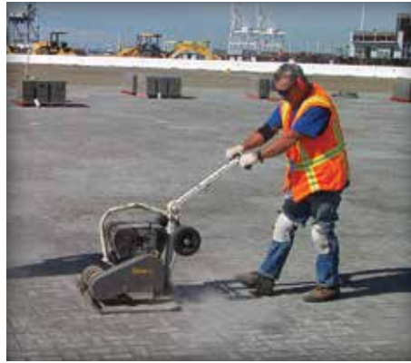
Figure 10. Initial compaction sets the concrete pavers into the bedding sand.
