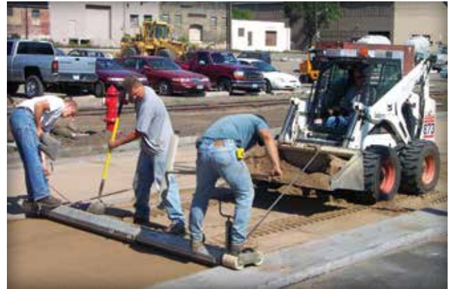
Figure 5. Mechanical screeding is the most efficient method of bedding sand installation
