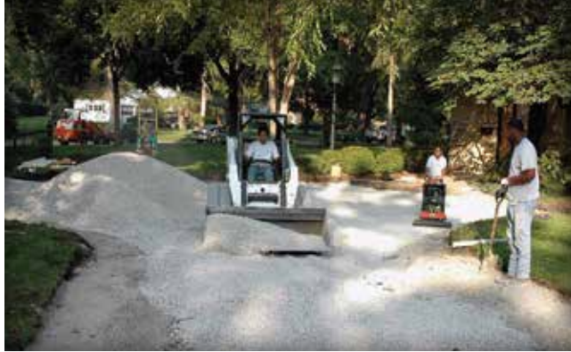
Figure 17. Perimeter berms made with dense-graded base are in place prior to placing open-graded aggregate in the driveway.
