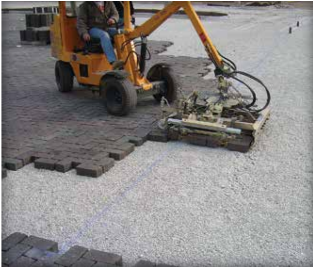
Figure 26 and 27. Mechanical equipment accelerated installation of a parking lot in Illinois and a street in Oregon.
