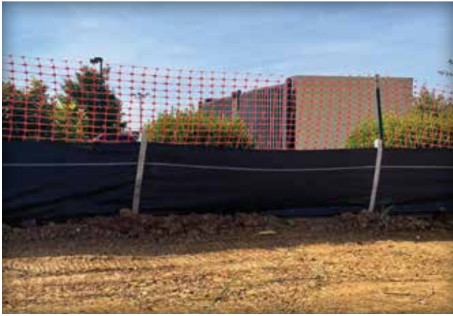
Figure 10. Typical silt fence application.
