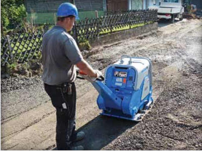
Figure 4. Base compaction with a reversible plate compactor.
