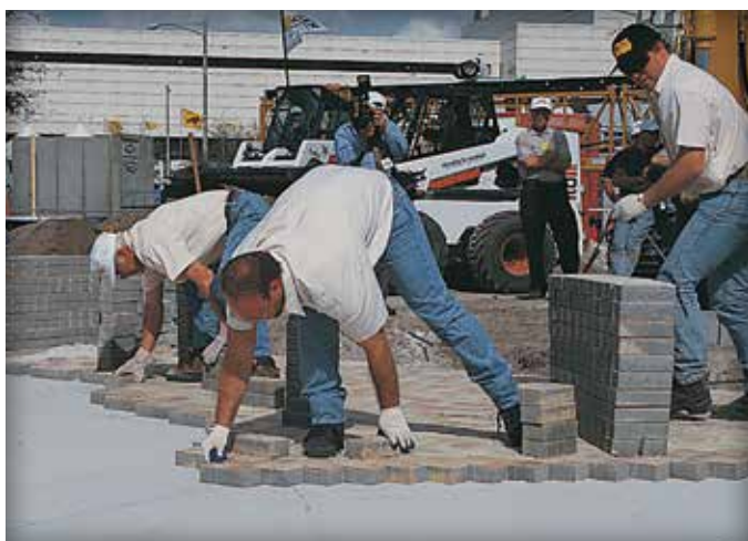
Figure 7. Placing the concrete pavers.
