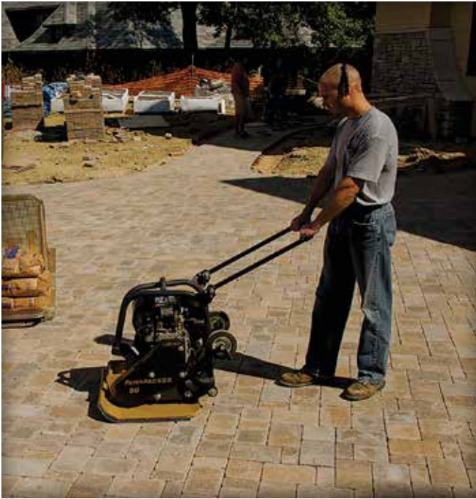
Figure 9. Compacting the pavers and bedding sand.
