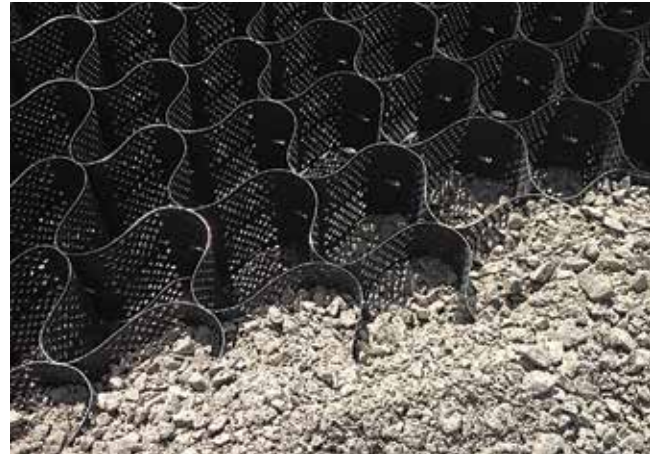
Figure 9. Geocells partly filled with aggregate
