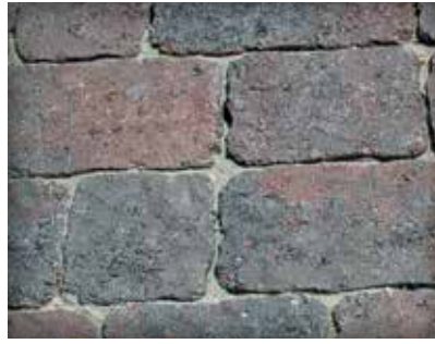
Figure 4. Liquid joint sand stabilizers can deepen the surface color slightly and they provide some surface sealing as well. Tumbled pavers shown here have wider joints than other shapes. These type of pavers can require stabilization of the joint sand.
