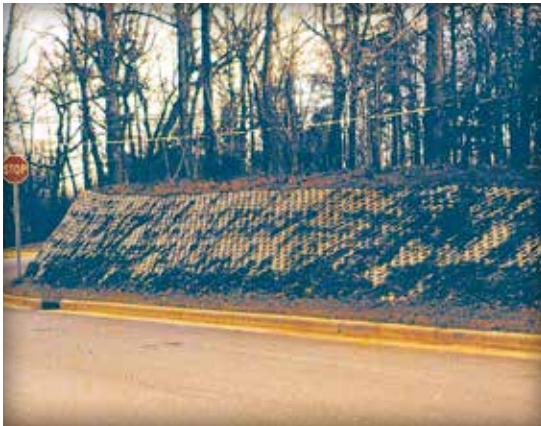
Figure 9. Embankment stabilization
