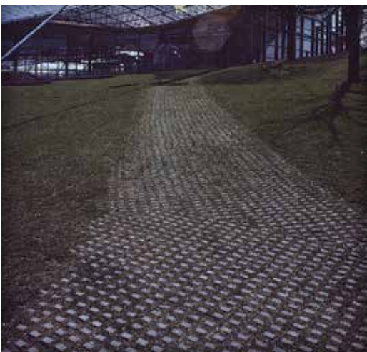
Figure 6. Service access lane
