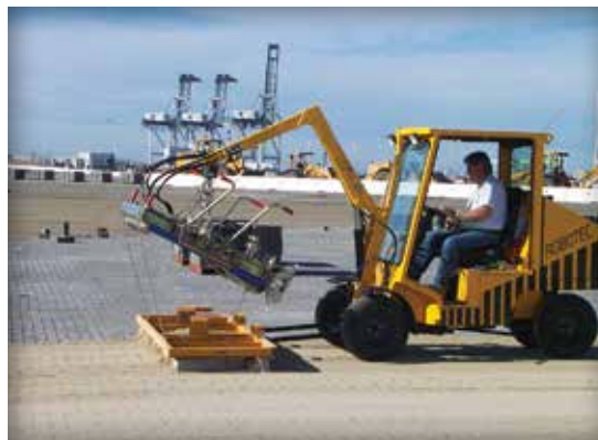
Figure 12. Sweeping jointing sand across the pavers is done after the initial compaction of the concrete pavers.
