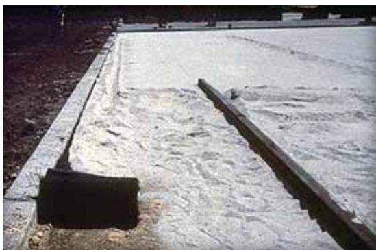
Figure 7. Woven geotextile used to contain bedding sand from migrating laterally. Visit [www.icpi.org](http://www.icpi.org) for detail drawings.
