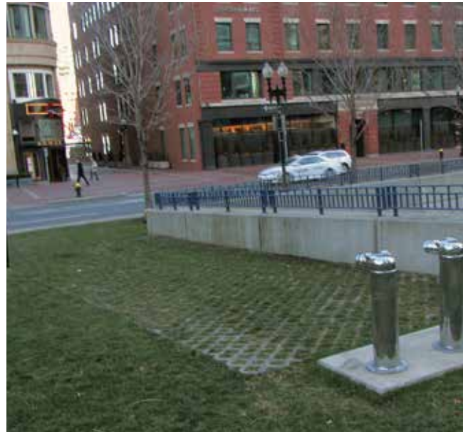
Figure 13. Concrete grid pavement typically reduces runoff in a manner similar to grassed surfaces.
