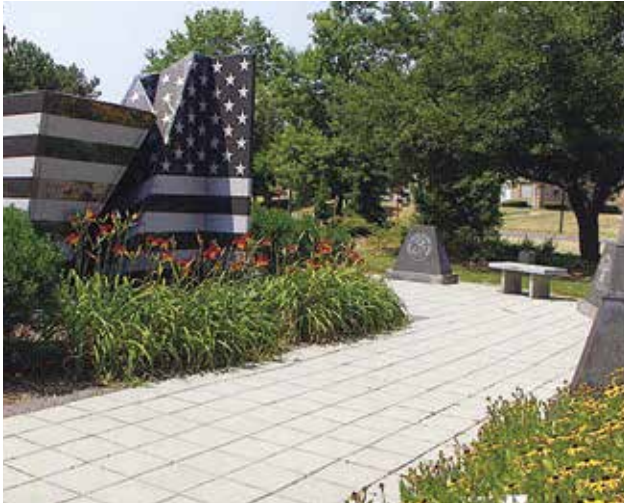
Figure 14. High SR paving slabs
