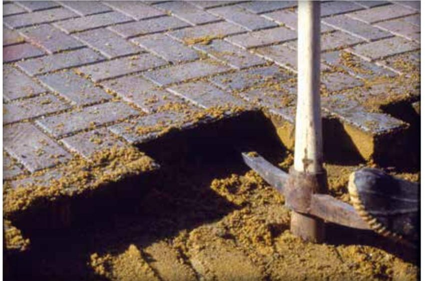
Figure 6. Prying out the remaining pavers
