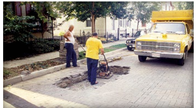
Figure 3. Compaction of the base
