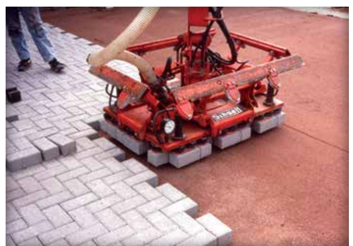
Figure 6. The vacuum head over the paver layer.
