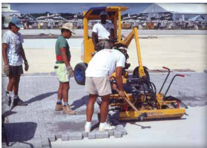
Figure 5. Motorized equipment with a hydraulic clamp.
