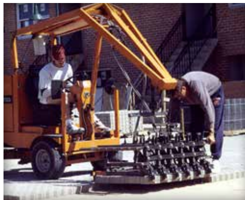
Figure 19. Mechanical equipment used to install concrete pavers on a roof deck.
