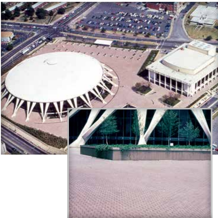
Figure 21. The plaza area around Scope Center in Norfolk, Virginia, (left) and one side of the Alamo Dome (right) in San Antonio, Texas, include roof plaza decks surfaced with concrete pavers.
