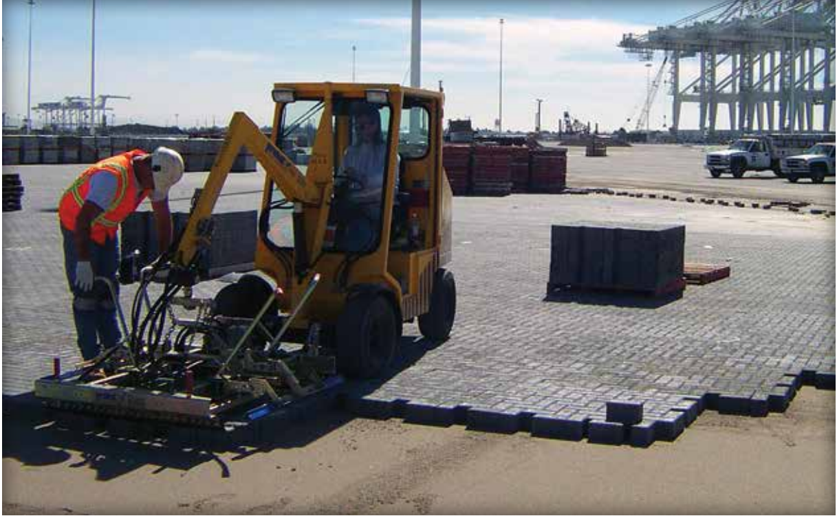
Figure 8. Mechanical installation equipment places concrete pavers rapidly.
