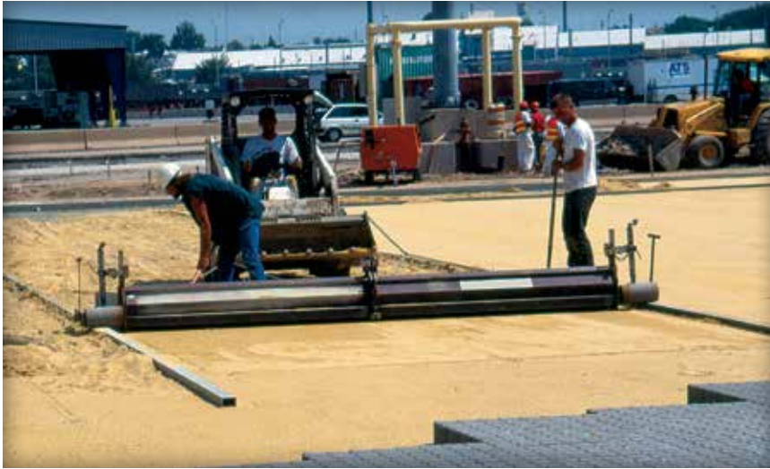
Figure 17. Powered screed bucket accelerates spreading of bedding sand. The width of the bucket can be adjusted.
