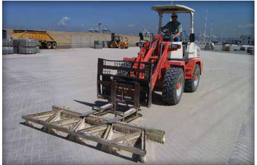
Figure 19. Broom attachments accelerate spreading and filling of joint sand.
