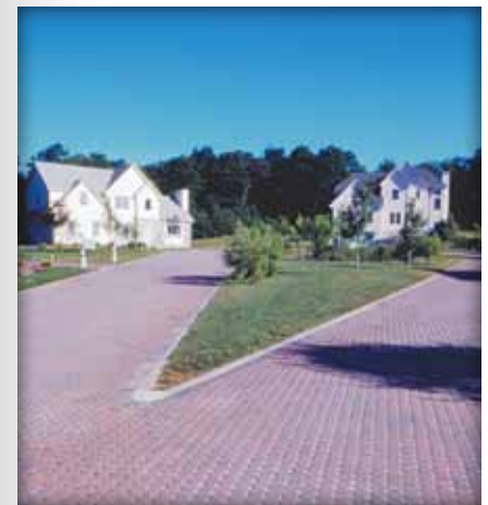
Rather than being paved, the center of the cul-de-sac in Glen Brook Green subdivision provides a bioswale to absorb runoff and overflow from the permeable pavement.
