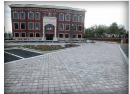
Runoff from the impervious asphalt surfaces is infiltrated into the PICP. The runoff is detained, filtered and infiltrated into the soil subgrade. Excess water is drained to storm sewers through perforated drain pipes in the base.
