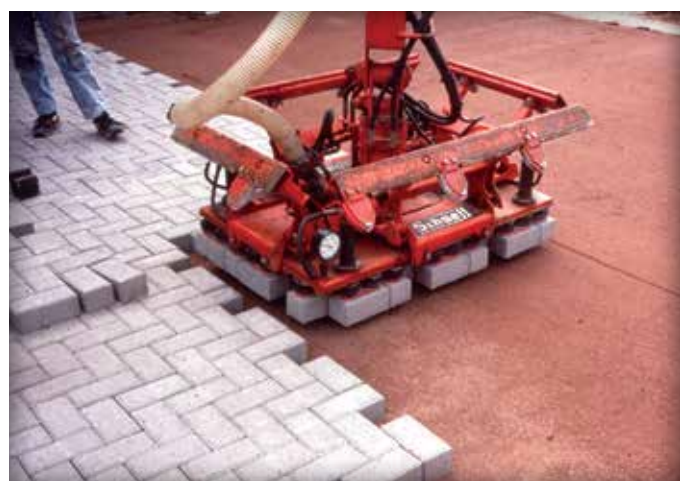
Figure 6. The vacuum head over the paver layer.
