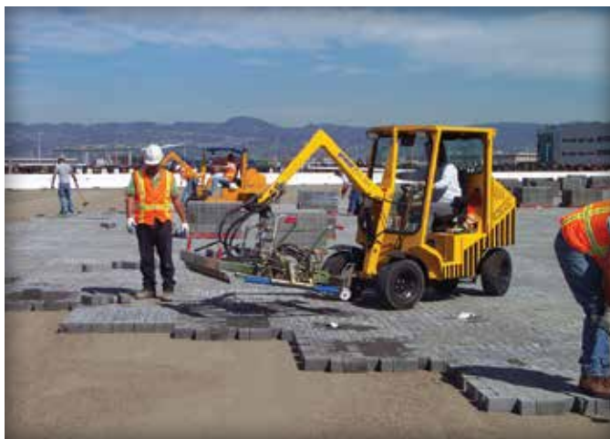
Figure 5. Motorized equipment with a hydraulic clamp.
