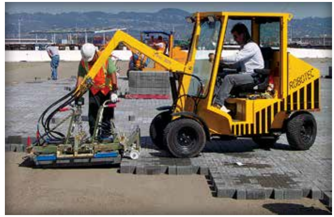
Figure 4. Hydraulic clamp picking up layer of pavers
