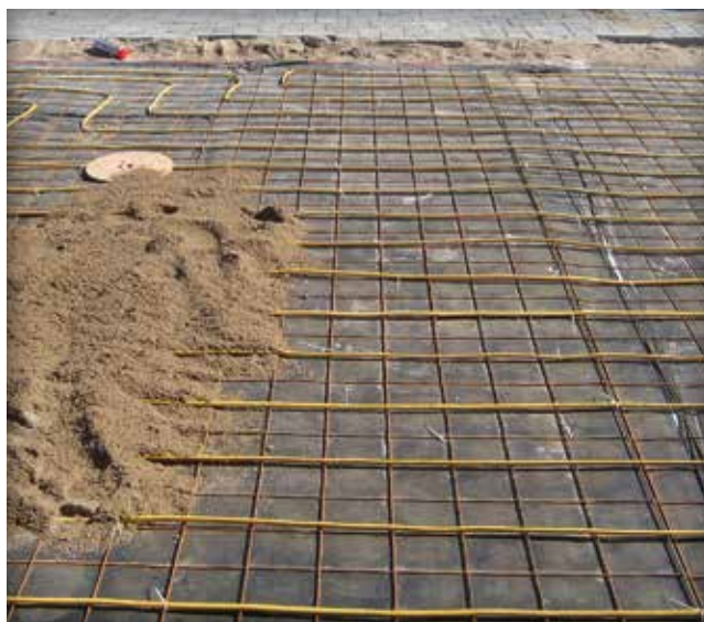
Figure 7. Spreading and screeding bedding sand must be done without moving or damaging pipes or wires for melting snow.
