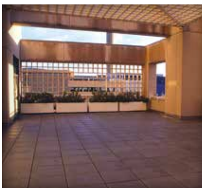
Figure 1. Concrete pavers provide a durable and attractive roof plaza deck surface. At left is the observation deck on the 86 th floor of Empire State Building in New York City. At center is a hotel plaza deck constructed with concrete paving slabs.
