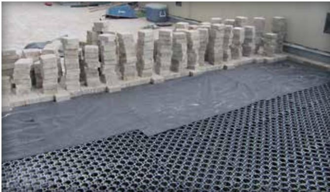
Figure 7. Concrete pavers on geotextile over plastic grids
