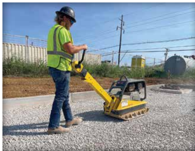
Figure 21. A larger reversible plate compactor is used to compact ASTM No. 57 stone base.
