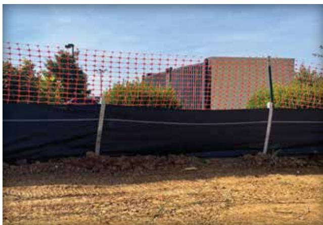
Figure 10. Typical silt fence application.
