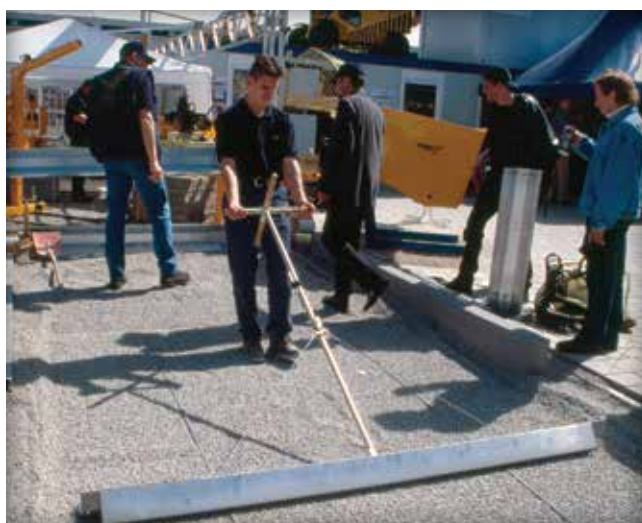
Figure 24. Manually screeding the No. 8 stone setting bed.
