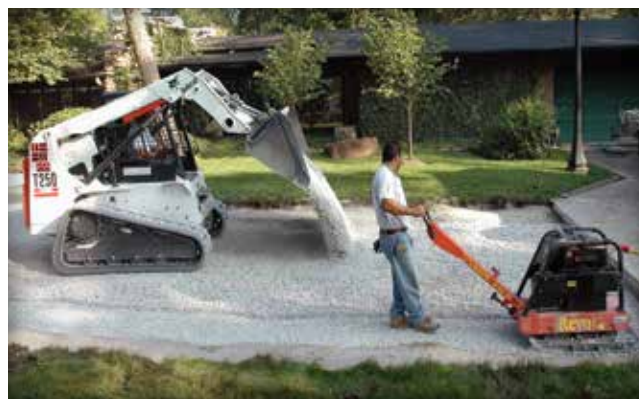
Figure 18. Compacting the berms along the perimeter and the PICP base
