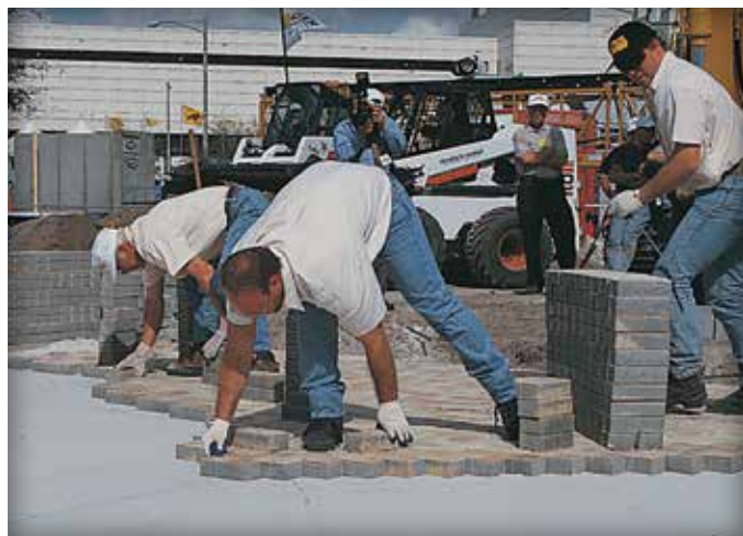
Figure 7. Placing the concrete pavers.
