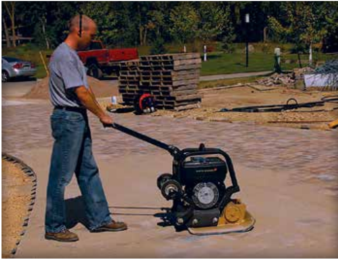
Figure 11. Vibrating sand into the joints.
