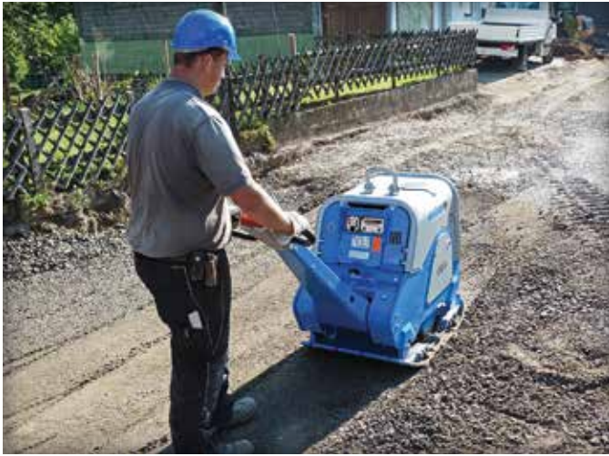
Figure 4. Base compaction with a reversible plate compactor.
