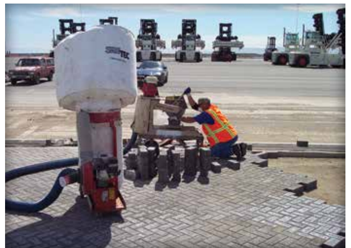
Figure 8. Saw cutting pavers.
