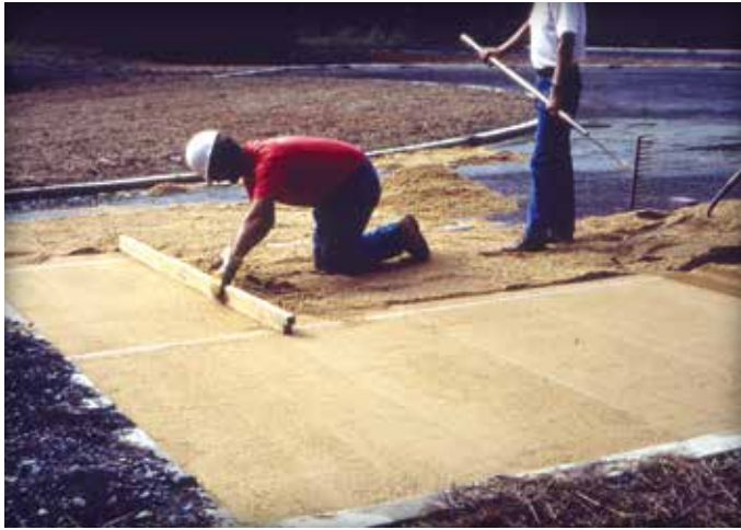
Figure 6a & 6b. Screeding the bedding sand.
