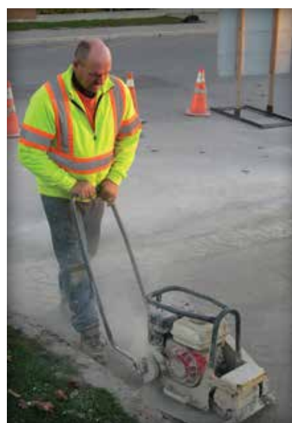
Figure 12. Once the pavers are in place, the joints are filled with dry joint sand and the surface is compacted.
