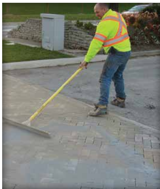
Figure 11. Sweeping in joint sand
