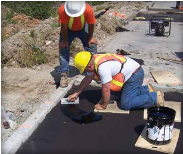
Figure 8. After the bitumen-sand mix cools, a 2% neoprene-asphalt adhesive is applied. The material can be trowel-applied as shown here. Adhesives with a lower viscosity can be spread with a squeegee.
