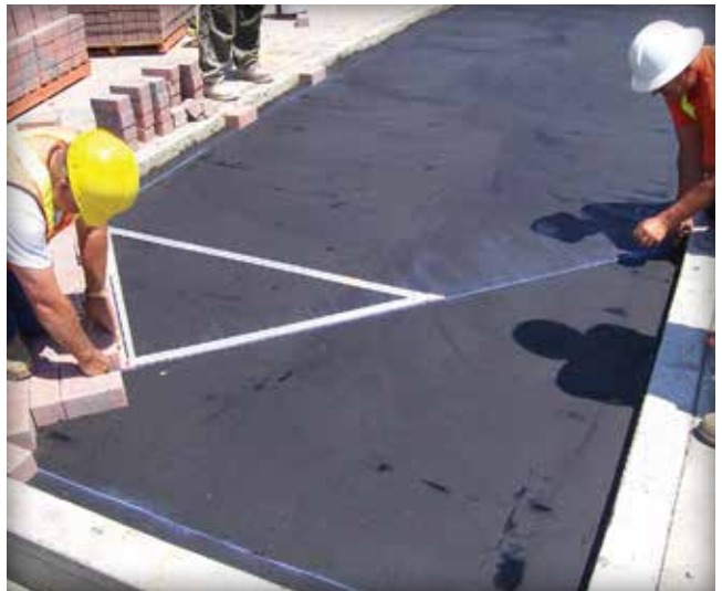
Figure 9. Perpendicular chalk lines are snapped and the pavers placed on the adhesive after the neoprene-asphalt adhesive dries (cloudy black surface).
