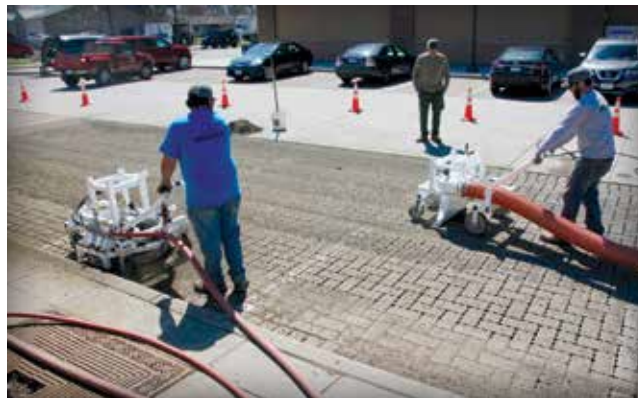
Figure 24. This equipment blows sediment and soiled aggregate from the joints and uses vacuum equipment to remove them.
