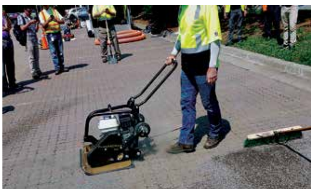
Figure 25. No matter the equipment used, after removing sediment soiled aggregate, clean aggregate is placed in the joints, the surface cleaned and compacted.
