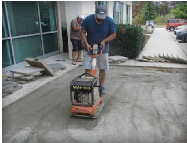
Figure 5. Precompacting the bedding sand
