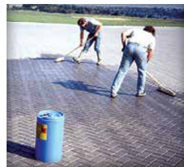
Figure 10. Urethane is applied with squeegees to stabilize joint sand between pavers on aircraft pavement.
