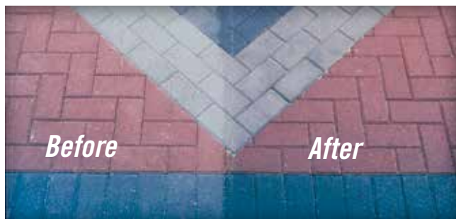
Figure 8. Before and after application of an acrylic sealer shows how it deepens the appearance of concrete pavers.
