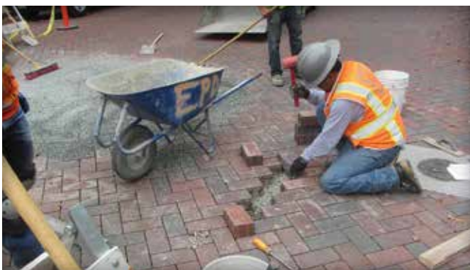
Figure 4. Reinstatement using the same pavers continues following the existing herringbone paving pattern.
