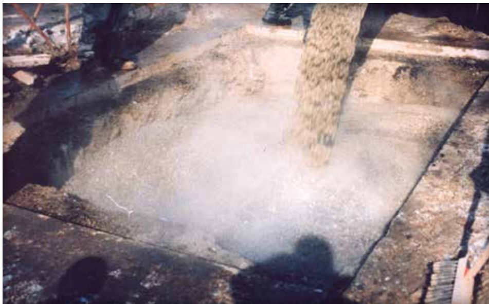
Figure 8. Low density concrete fill (unshrinkable fill) poured into a utility trench from a ready-mix concrete truck.
