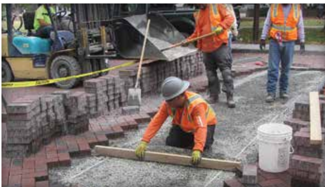
Figure 2. After compaction of the base, bedding material is screeded.
