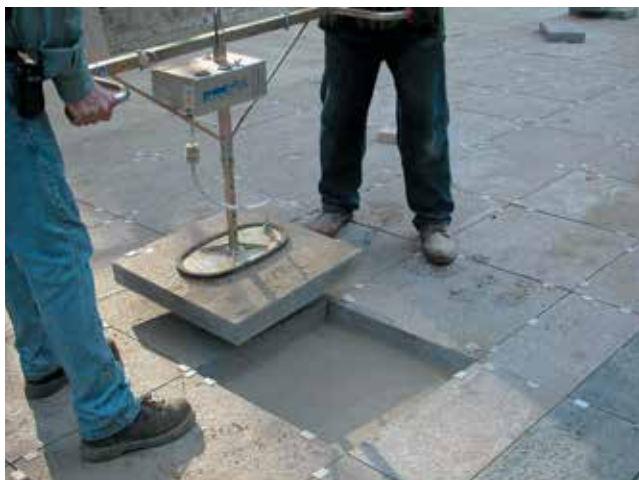
Figure 14. Two-person vacuum lift for paving slabs
