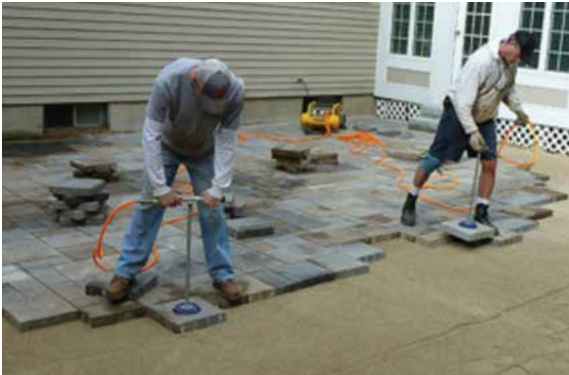
Figure 16. Using vacuum equipment to install paving slabs in a residential application
