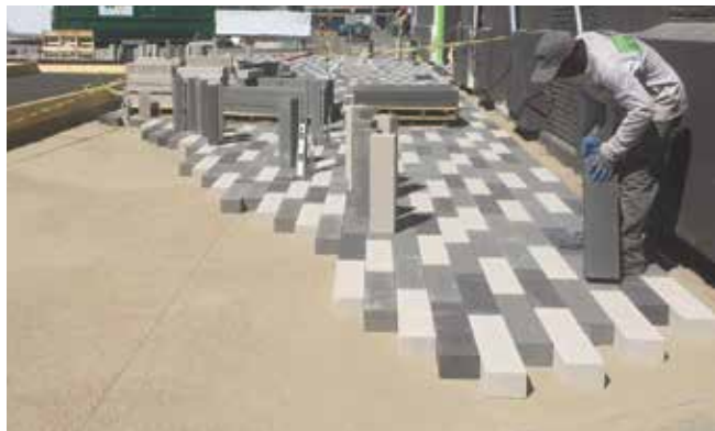
Figure 6. Installing planks on uncompacted bedding sand.
