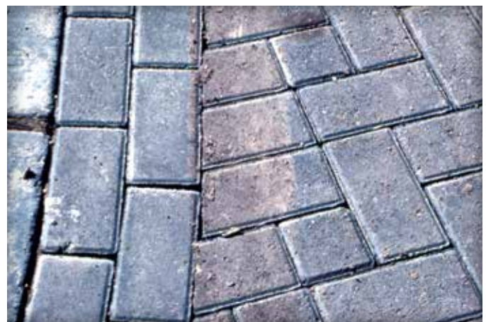
Figure 14. A double row of manually placed pavers along a curb or building provides maneuvering space for the mechanical installation clamp.
