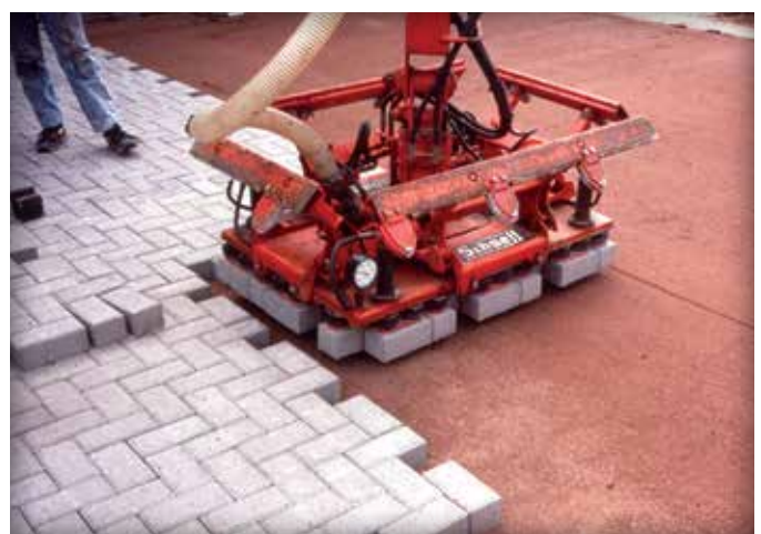
Figure 6. The vacuum head over the paver layer.
