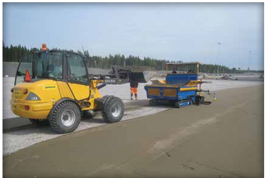
Figure 18. A screeding machine can evenly and rapidly spread bedding sand.
