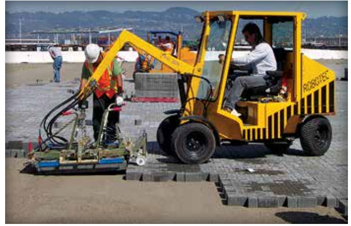
Figure 4. Hydraulic clamp picking up layer of pavers
