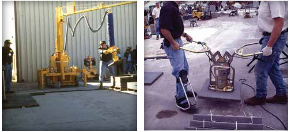
Figure 21. Vacuum assisted mechanical equipment for installing paving slabs.
