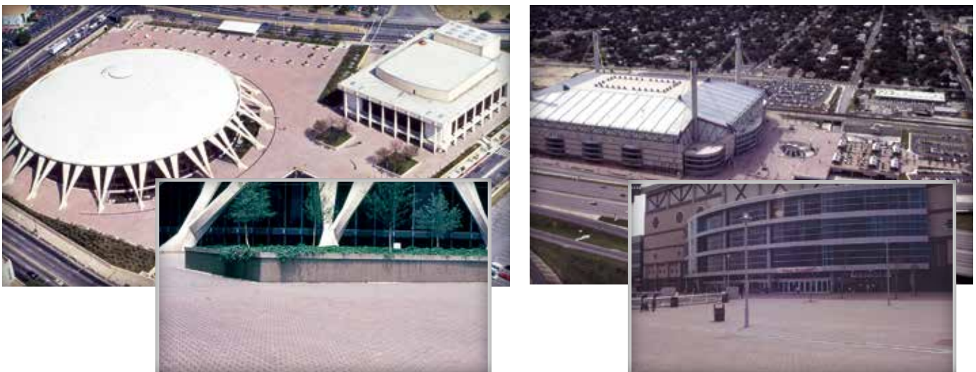
Figure 22. The plaza area around Scope Center in Norfolk, Virginia, (left) and one side of the Alamo Dome (right) in San Antonio, Texas, include roof plaza decks surfaced with concrete pavers.
