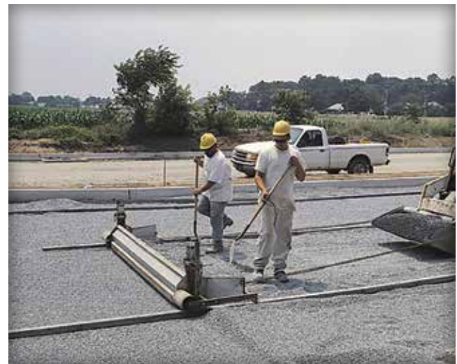
Figure 25. A screed beam pulled by equipment can be more efficient and productive.
