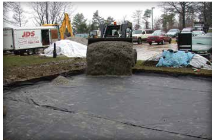
Figure 3. Application of the geotextile under aggregate base.
