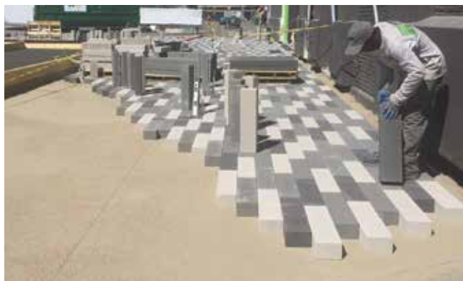
Figure 6. Installing planks on uncompacted bedding sand.
