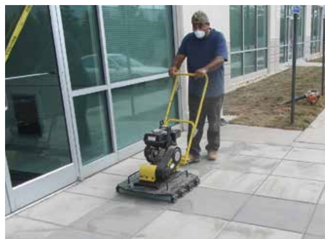
Figure 19. Compacting paving slabs with a roller attachment on a plate compactor
