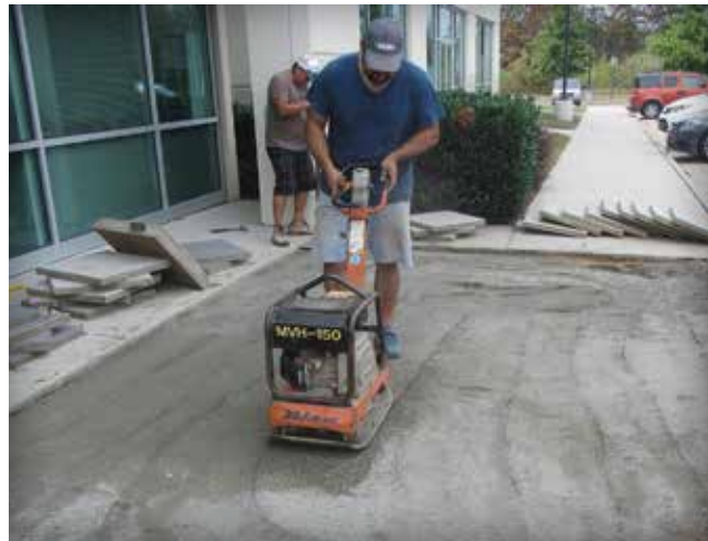
Figure 5. Precompacting the bedding sand
