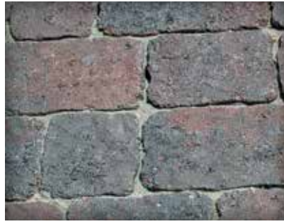
Figure 4. Liquid joint sand stabilizers can deepen the surface color slightly and they provide some surface sealing as well. Tumbled pavers shown here have wider joints than other shapes. These type of pavers can require stabilization of the joint sand.
