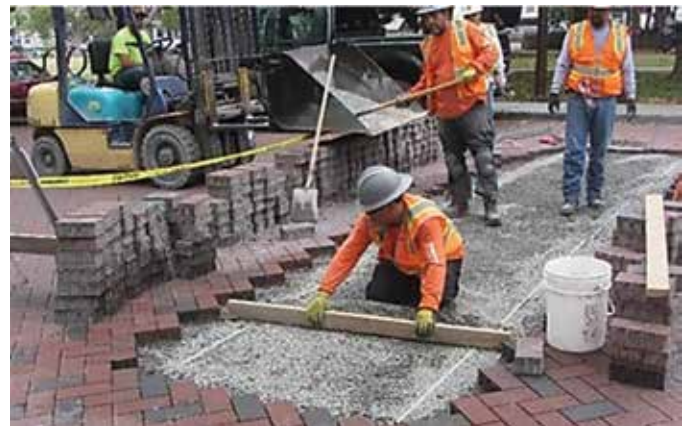
Figure 39. Alternately screed bar can be placed on the re-established base.
