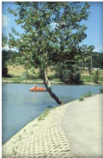
Figure 4. Lakeside stabilization
