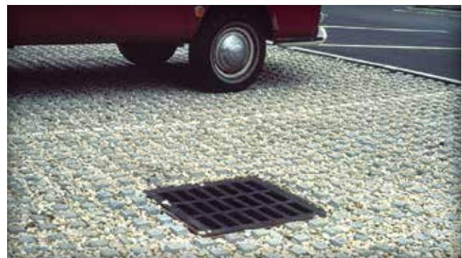
Figure 16. Concrete grids with aggregate in the openings
