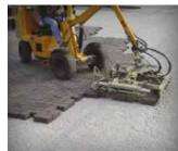
Mechanical installation equipment accelerates construction; typical 5,000 sf (500  $m^2$ )/machine/day. After placement, joints and/or openings filled with small aggregate and pavers are compacted.
