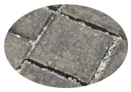
Permeable joint material consisting of small aggregates allows infiltration of stormwater.
