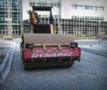
Base construction uses locally available materials. Pavers are delivered ready to place, joints filled, compacted and ready for traffic.
