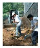
Site layout and excavation: The layout of interlocking concrete pavement translates the drawing into reality. In addition to knowing the size of the pavement and excavated area, the layout tells the contractor the sequence of job functions and crew involvement. Considering all factors in advance such as material storage and paving direction helps ensure a smooth operation.
