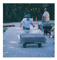
Paver compaction and Joint Sand: Pavers are first compacted without joint sand to create initial interlock. After this is complete, dry joint sand is spread and swept and the pavers compacted again until the joints are completely full. Following compaction and removal of excess sand, you and the contractor should inspect the pavement together to ensure satisfaction.
