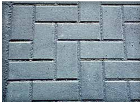
Figure 7. A close-up of the concrete paver surface at the PTI test track.
