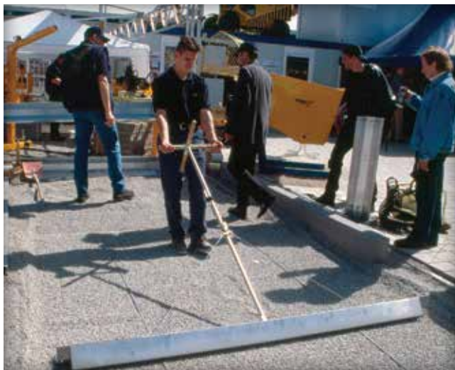
Figure 24. Manually screeding the No. 8 stone setting bed.
