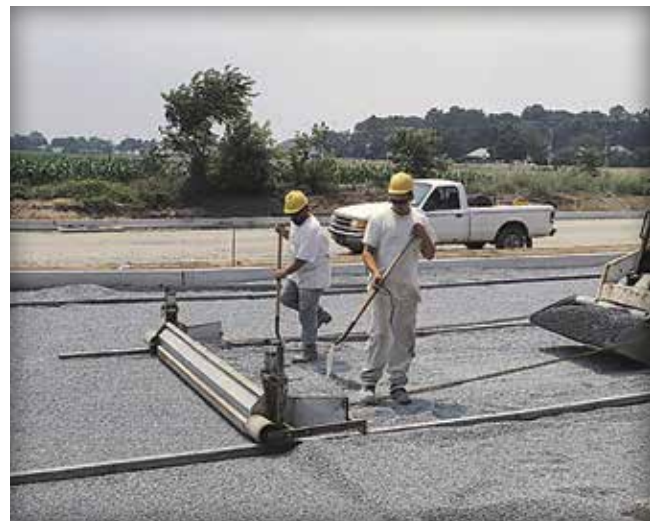
Figure 25. A screed beam pulled by equipment can be more efficient and productive.
