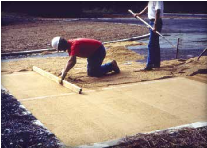
Figure 6a & 6b. Screeding the bedding sand.
