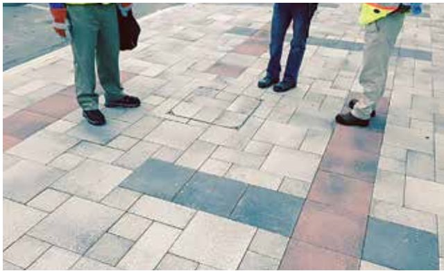
Figure 27. Example of a utility cover that does not fit neatly into the paving pattern.
