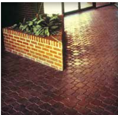
Figure 1. Many sealers enhance the appearance of concrete pavers and protect against staining.
